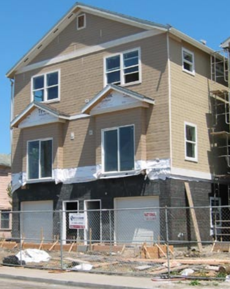
OCHI's multi-story manufactured townhomes under construction at Linden A in Oakland.
