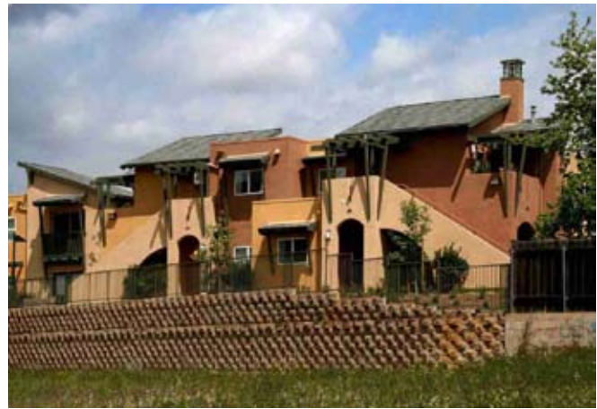
Solara, a 56-unit affordable housing project in San Diego County, is one of the rare projects that is using PV panels to power all residential and common areas, including a computer learning center. Developed by CommunityHousingWorks and opened in 2007, Solara financed the panels using federal investment tax credits and received a rebate on the cost of the panels from the California Energy Commission.
