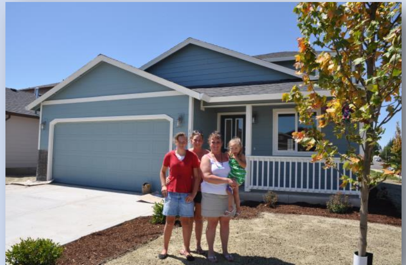
Self-help housing in Gervais, Oregon, built with technical assistance from Community Homebuilders.
