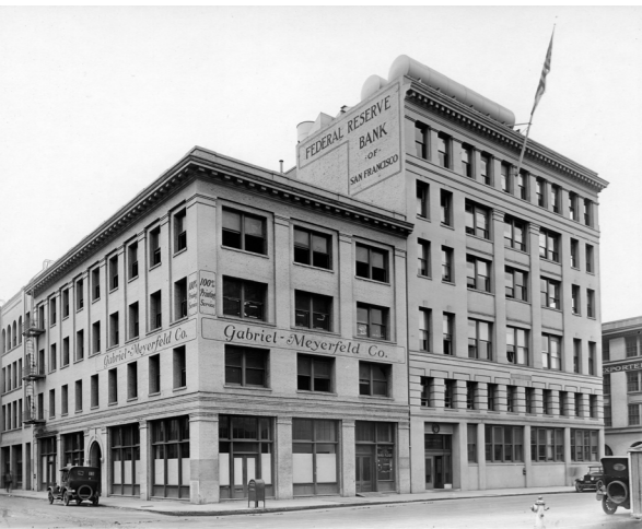
San Francisco Fed Headquarters 315 Battery Street 1918 – 1923
