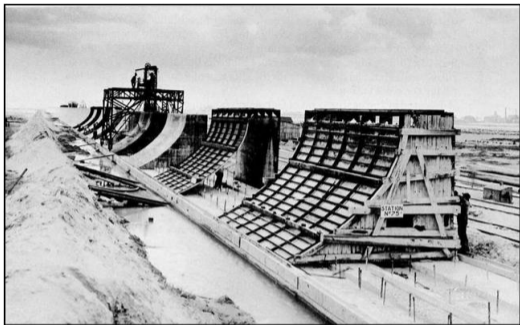
Figure: Construction of old Galveston, TX sea wall
