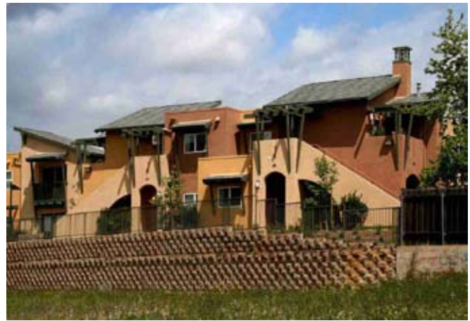
Solara, a 56-unit affordable housing project in San Diego County, is one of the rare projects that is using PV panels to power all residential and common areas, including a computer learning center. Developed by CommunityHousingWorks and opened in 2007, Solara financed the panels using federal investment tax credits and received a rebate on the cost of the panels from the California Energy Commission.
